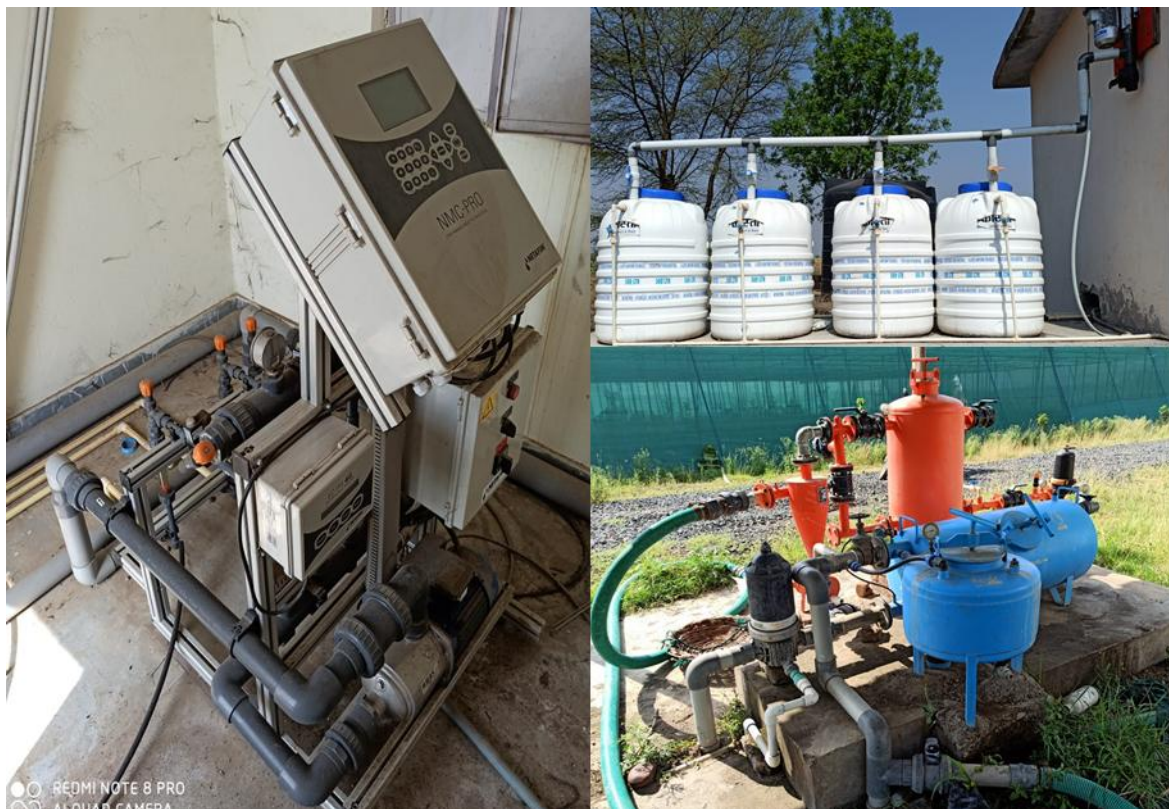
Figure 2 Drip Fertigation System
