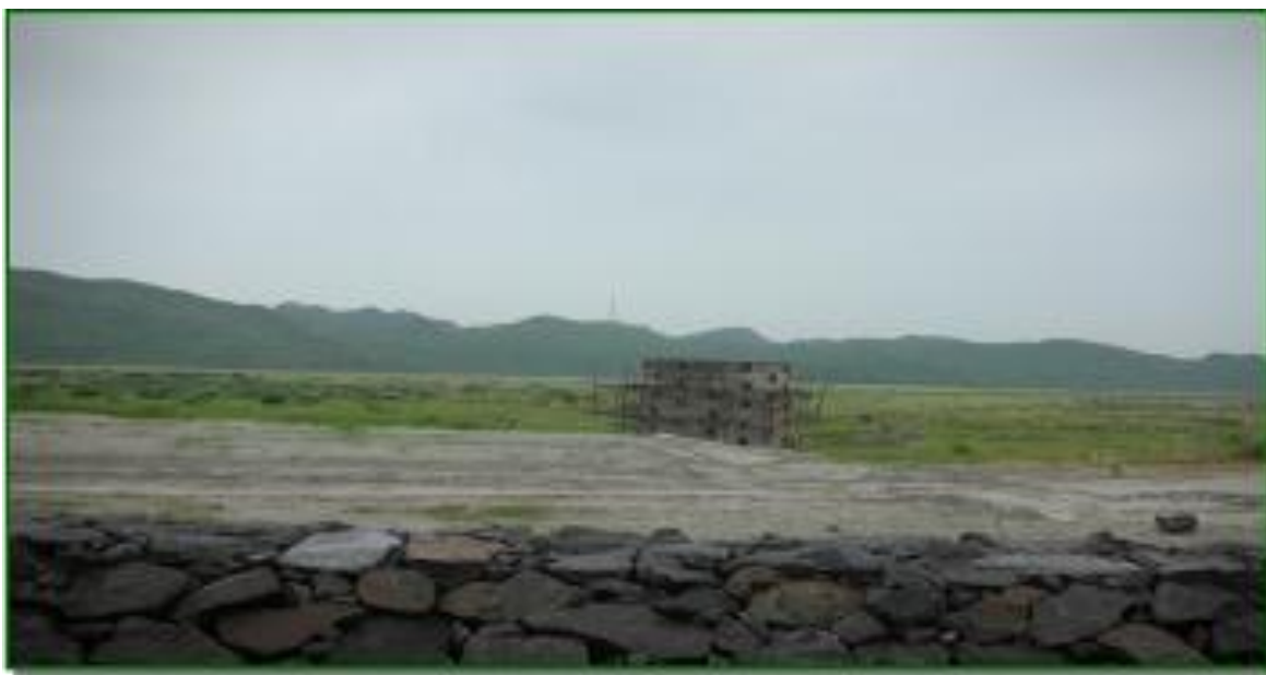
Figure 1 Ash pond Located at 7 km distance from NTTPS with Decantation filter in the Center of the pond
