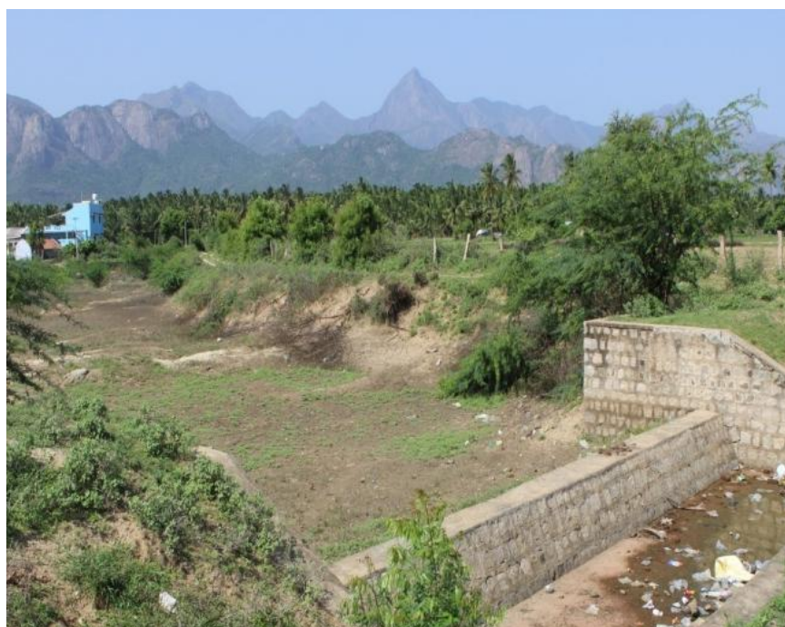
Figure 3 Check dam without water
