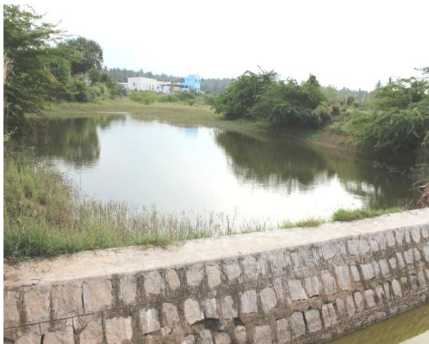
Figure 2 Check dam filled with water
