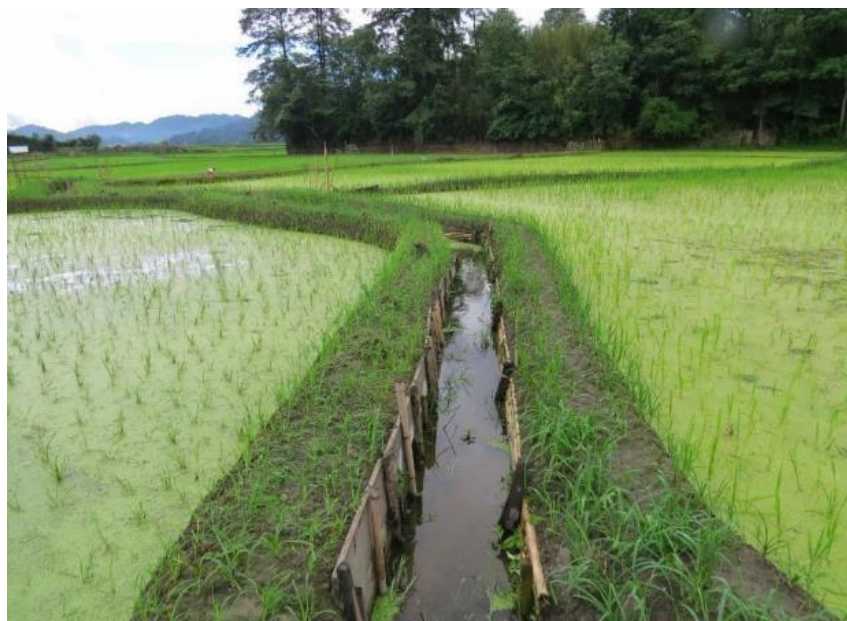
Figure 5 A typical water conservation structure designed for dual purpose (growing crops and pisciculture along the channels) ( http://www.cprecevis.nic.in/ ) [10]
